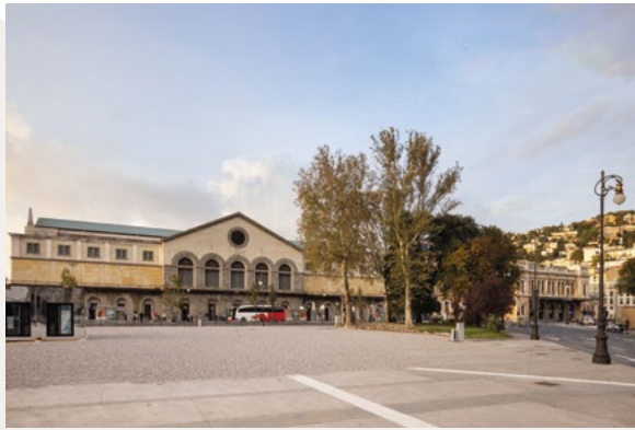
1 Silos e Stazione di Trieste Silos in tržaška železniška postaja Silos and Trieste central railway station
